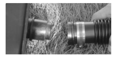
8. Connect provided flex hose to the end labeled "To Pool" and the opposite end to the return fitting. Tighten hose clamp with screwdriver.
