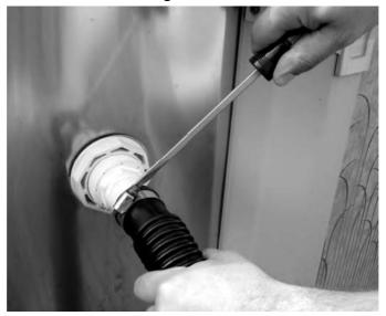
7. Take the hose end removed from pool return and connect to hose adaptor attached to the header. Tighten hose clamp with screwdriver.
