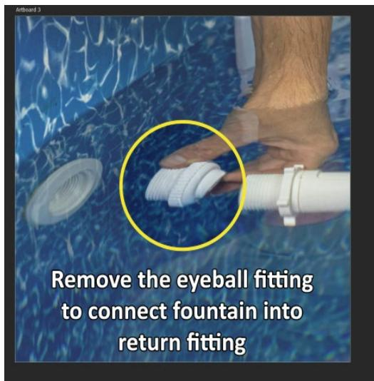
You can now thread the fountain fitting into the return. Adjust flow valve to desired height for your pool after you turn pump back on.
