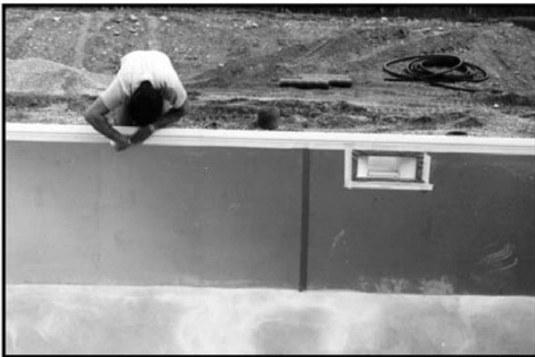
Tape off vertical wall seams.
