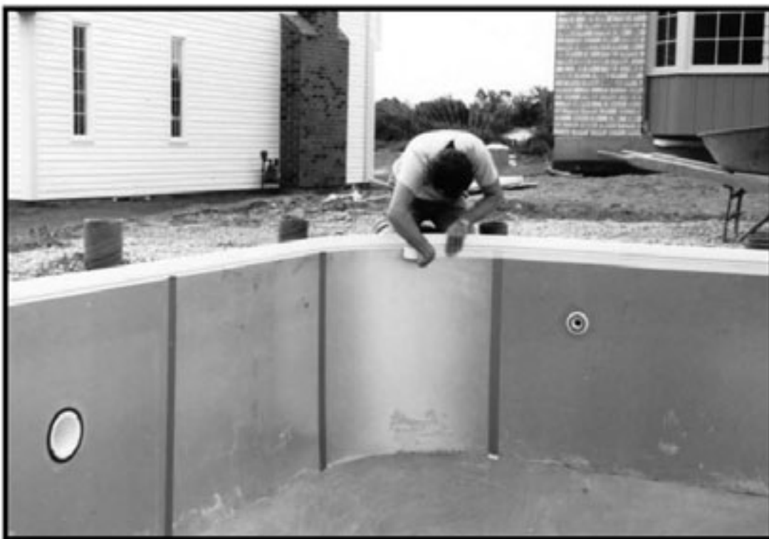
Tape around the perimeter of the coping.
