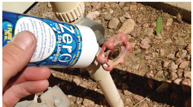
Releases seized ball and backwash valves without breaking them.
