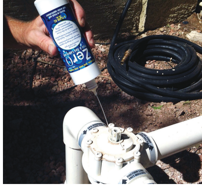
ZerO will go places traditional lube cannot. Without disassembling fixtures, you can reach problem area O-rings to troubleshoot or perform preventative maintenance.
