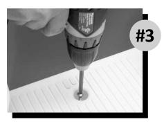
Check to make sure the hole locations in the platform are clear of pool wall and supports. Drill two 5/16" holes through the Platform and pool top ledge. Fasten the ladder platform to the pool ledge using two ½"-20 x 3-½" bolts, ½"-20 hex nuts.
