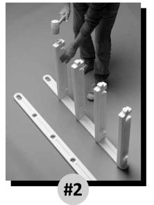
Using a rubber mallet, tap the Swing-up Treads into place.
