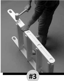
Place the other Swing-up Rail over the tabs of the Swing-up Treads, making sure the pegs align. Tap into place using rubber mallet. Set this assembly aside.
