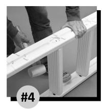
Place the opposite Side Rail assembly on top of the Fixed Ladder Treads so that the notches and tabs align and tap it into place. Placing your foot on the Side Rail to hold it steady, use the rubber mallet to tap down the Fixed Ladder Treads until they are firmly seated into both Side Rails.
