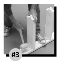
Placing your foot on the Side Rail to hold it steady, use the rubber mallet to tap down the Fixed Ladder Treads until they are firmly seated in the Side Rail.
