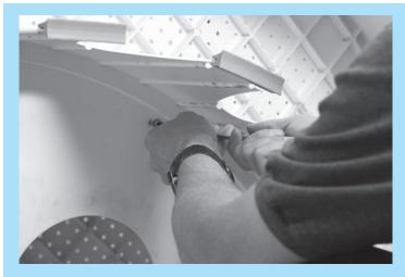
Once the 9 holes are lined up secure the base step to the step assembly until all 9 screws are in place along with the stainless steel washers. Be sure to hand tighten only using the screw driver that comes with the step.
